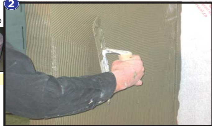
Apply membrane, smooth out with trowel
