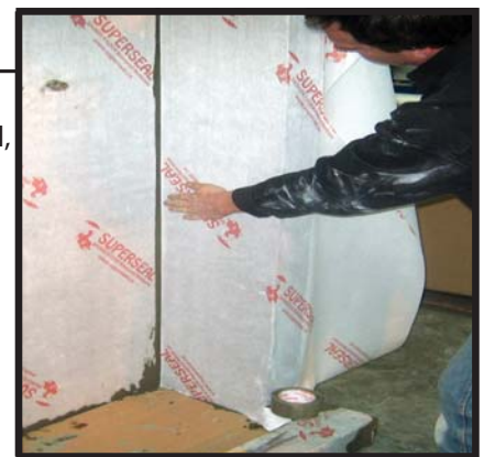
Apply membrane, smooth out with trowel
