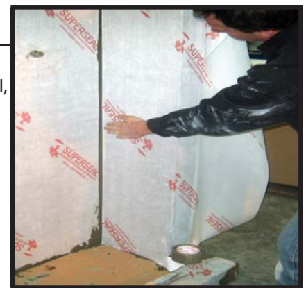
Apply membrane, smooth out with trowel
