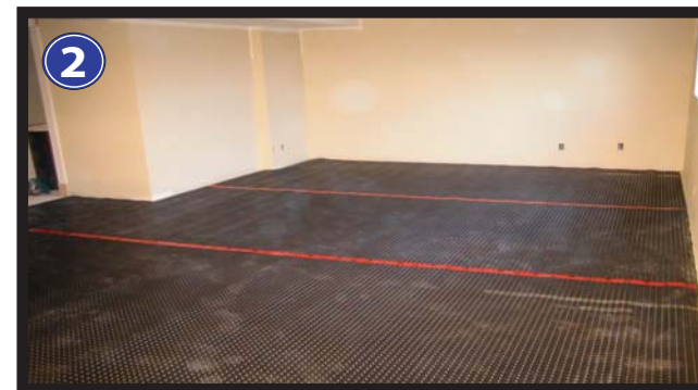
3 10 mil (3/8") or thicker laminate flooring can be installed directly on top of membrane.
