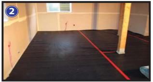
Butt edges together and tape seams with vapor barrier tape
