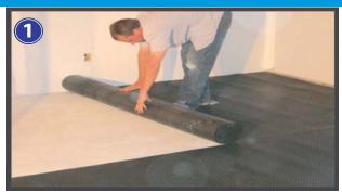
Unroll All-In-One and cut to fit. Leave a 1/4" gap around walls stairs and supports
