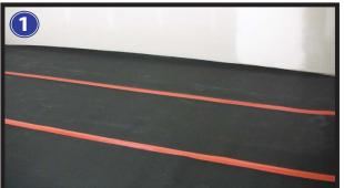
Unroll membrane and cut to fit. Flip membrane over, butt edges together and tape the seams.
